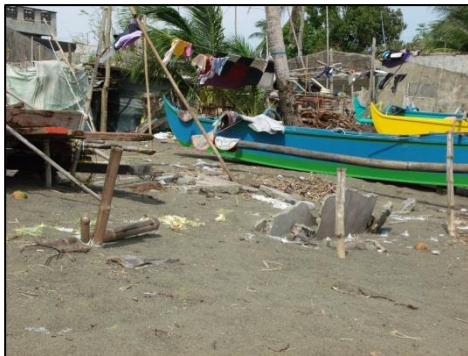
Fig. 5. House destroyed along the shoreline of Brgy. Naulo.
